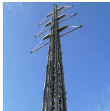
Figure B4.2: The new “VITRUVIO“ lattice tower in shape of a monopole tower
