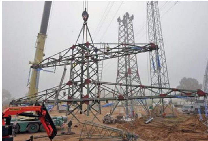
Figure B3.1: Modular construction with bolted connections
