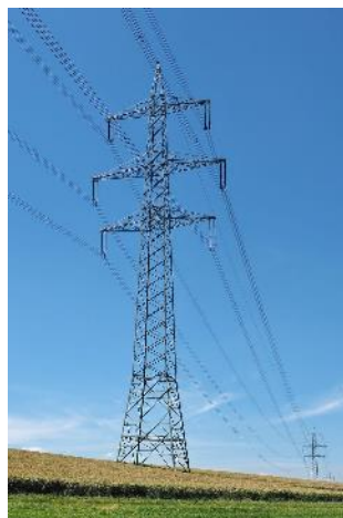
Figure B3.16: Barrel tower
