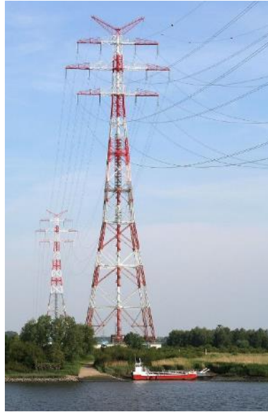
Figure B1.2: Elbe Crossing 2 transmission towers
