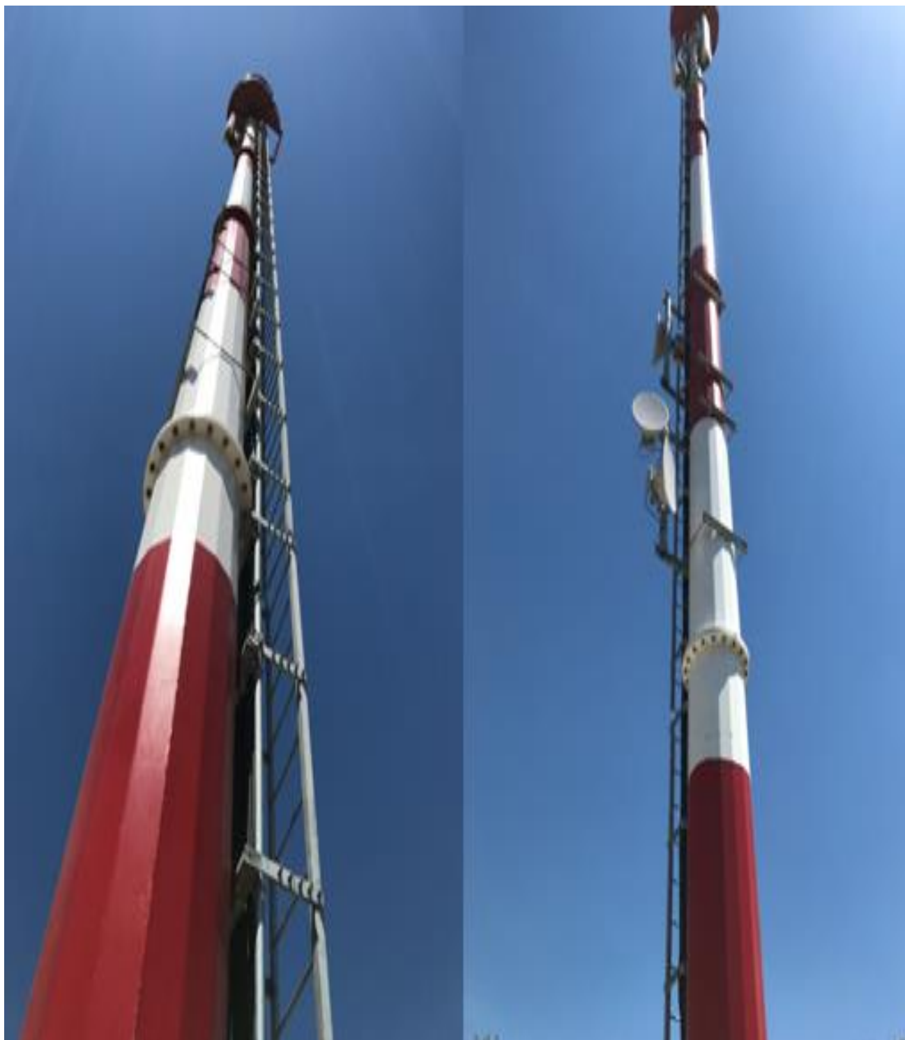
Figure A4.1: Polygonal Towers
