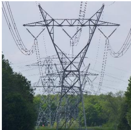
Figure B3.12: Delta tower with one circuit
