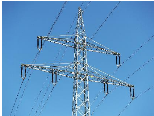
Figure B3.8: Cross arms of a lattice tower
