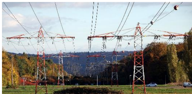
Figure B3.14: Single plane towers at the airport of Karlsruhe, Germany
