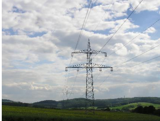
Figure B3.15: Danube tower
