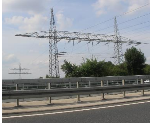
Figure B3.11: Anchor portal tower
